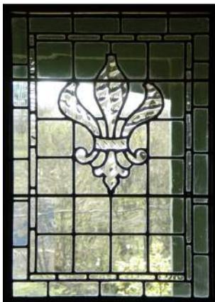
Now let us look at the windows at St Mary's. The first window is in the entrance door. It includes textured glass, which is machine made, although I confess I don't know how. The central panel is surrounded by a double border of straight strips of glass. Such a border is common in stained glass windows and I have been told that the idea was that if anything was going to be broken during handling it would be an easy-to-replace strip rather than a costly painted piece.
